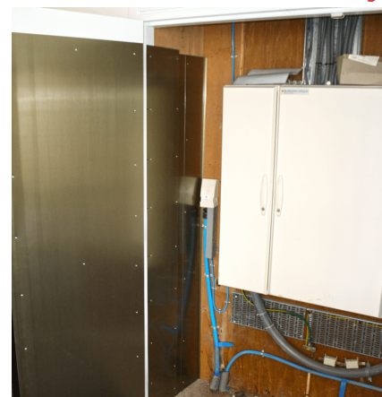
Example of a Mu-ferro cable trunking in a meter box. The walls and door are equipped with mu-ferro magnetic shielding as well
