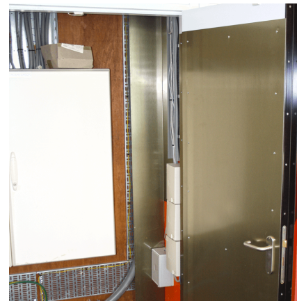
Example of a Mu-ferro cable trunking in a meter box. The doors are also equipped with a mu-ferro magnetic shielding
