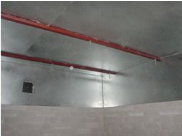
MuFerro 6800 ceiling umbrella construction
